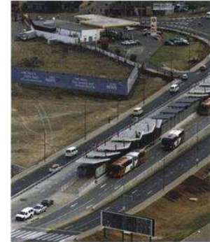
ABOVE A completed BRT station
