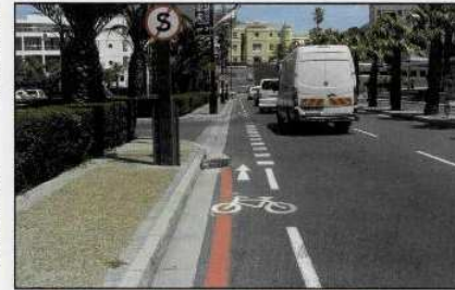
Above: Cycleway under construction running parallel to the IRT route Below: Cycle lane painted alongside the raised pedestrian pathway
