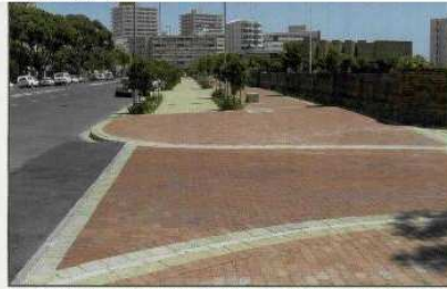
Pedestrian and cycle surfaces continue over Bellmouth to reduce the speed of turning vehicles and thereby give right of way to pedestrians and cyclists
