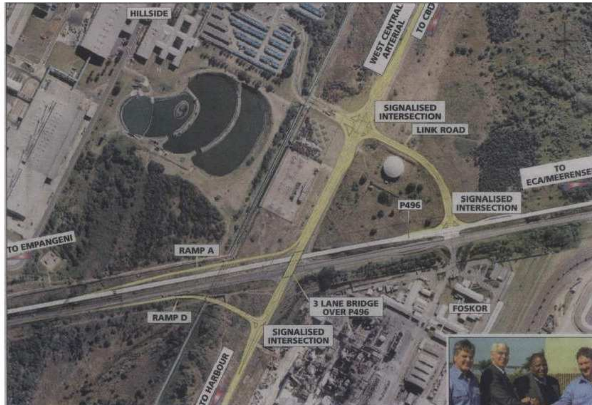
The new West Central Arterial and John Ross Highway intersection in Richards Bay where an overpass and new link road will improve road safety. Inset: Marking the start of the R75 million project were, from left, BHP Billiton Aluminium project director Danie Murray, uThungulu District mayor Stan Larkan, City of uMhlatuze mayor Zakhele Mnqayi and Aluminium SA asset president Gustav Griessel.
