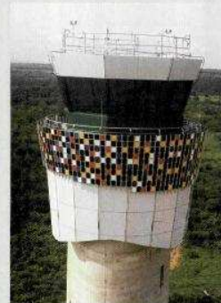
The completed control tower.
