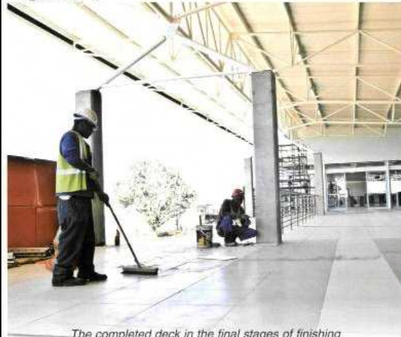
The completed deck in the final stages of finishing
