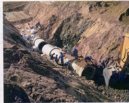
HELDERBERG COASTAL SEWERAGE
