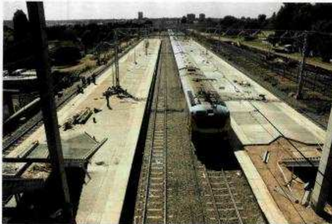
ABOVE LEFT A train passes under the 'in construction' station
