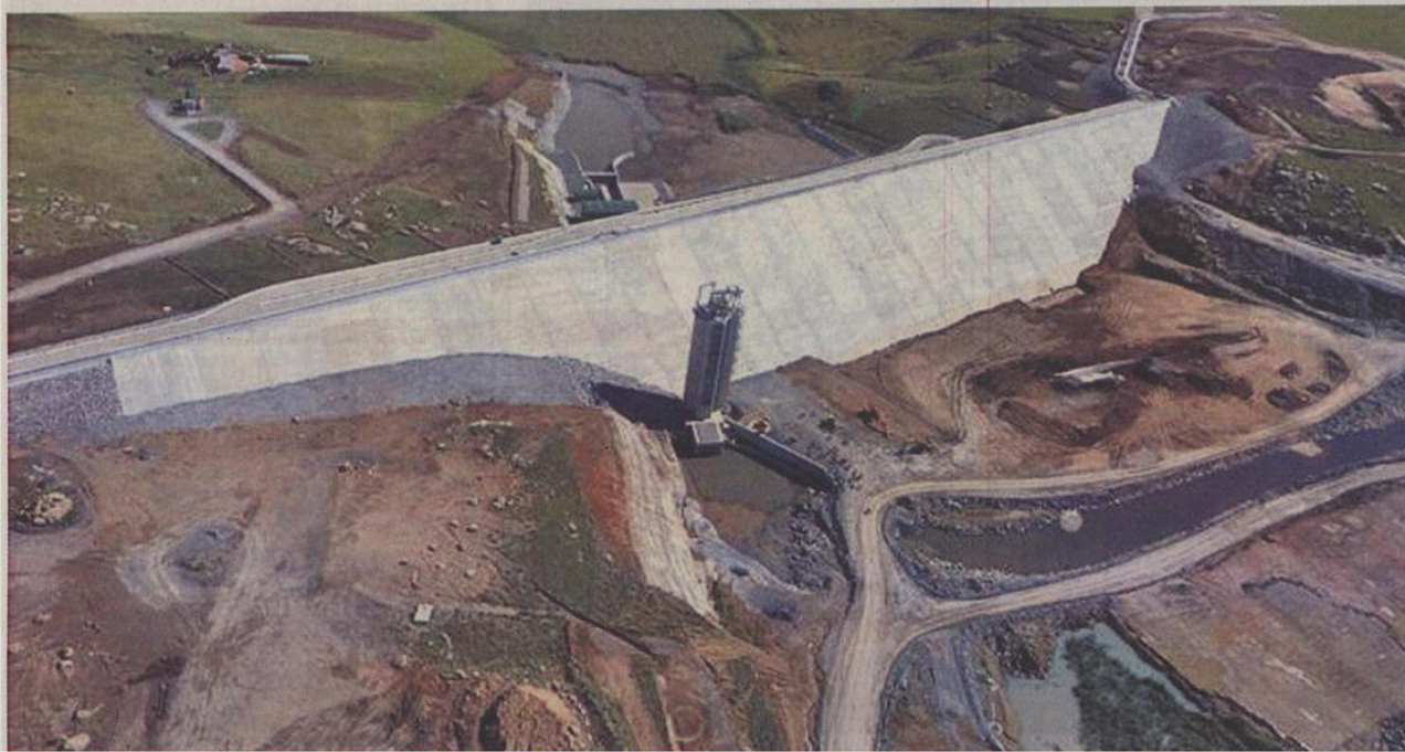
DAM FINE: The Cesa Award for Engineering Excellence on projects with a value greater than R250-million was won by the Braamhoek Consultants Joint Venture, comprising GIBB, Knight Piésold and SSI Engineers and Environmental Consultants, for the Bedford Dam-Ingula Pump Storage Scheme for Eskom
