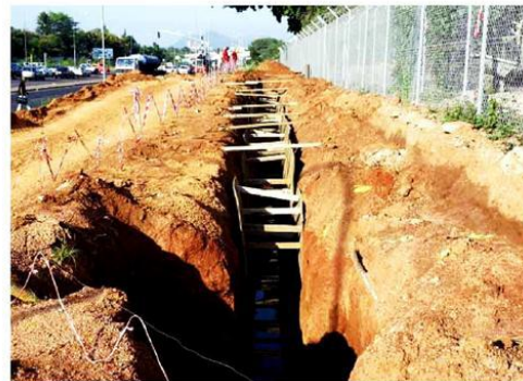
Trench shoring to prevent collapse
